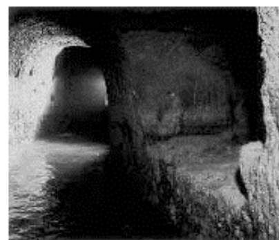
Figure 3. Main tunnel (left) and an adit (right)
