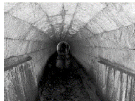
Figure 7. Tunnel by piling-stones with an arch type
