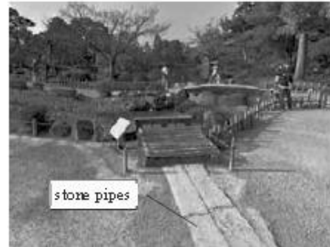
Figure 15. Remains of stone pipes near the final point D of the inlet of the inverted siphon in Kenrokuen garden
